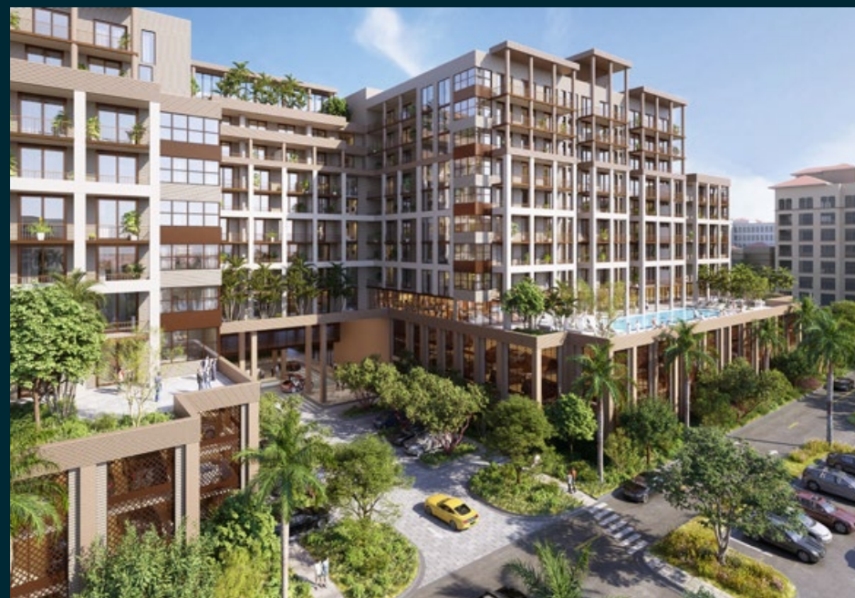
SE 4TH STREET // BOCA RATON
